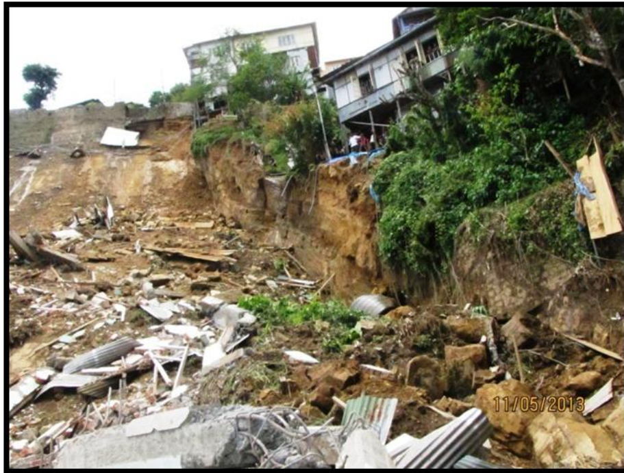
Figure 6. Photograph showing the rapture surface, crown and minor scraps.
