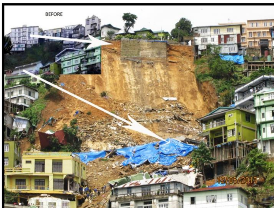
Figure 3. Laipuitlang Rockslide view from Ramhlun Venglai.
